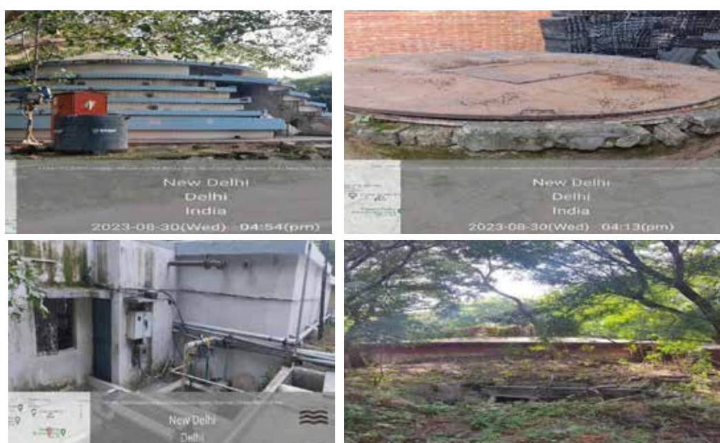
Water Storage Tanks at IGNOU
